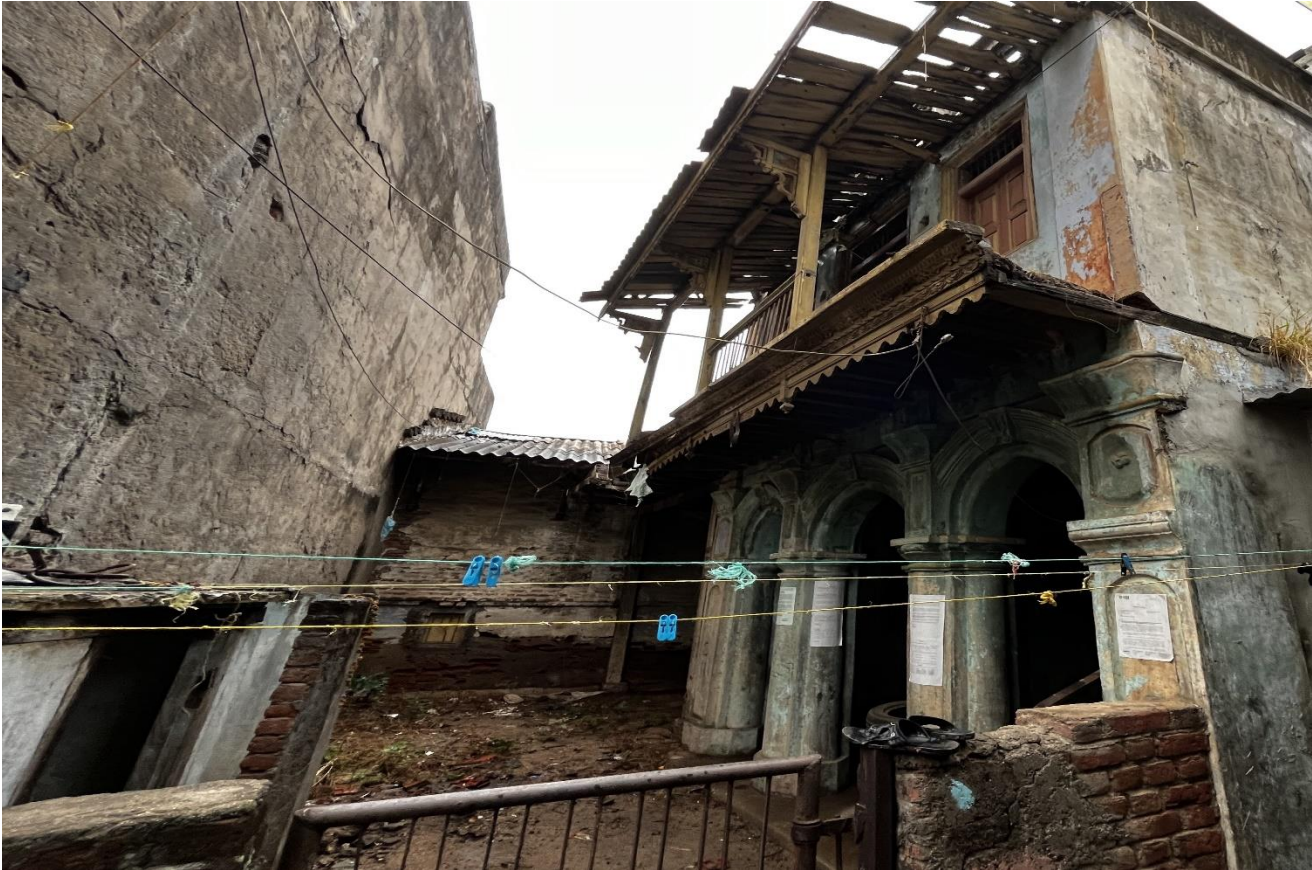
Residential house at Baneida :-
